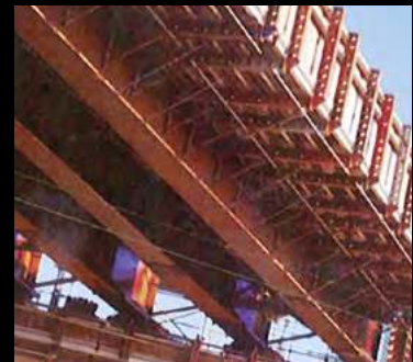
FARRRS bridge beams spanning the East Coast Mainline
